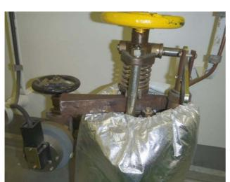
Quick Closing Valve gagged with steel wedge
