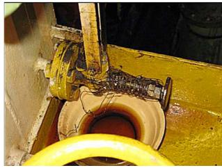
Self Closing Valve gagged with wire
