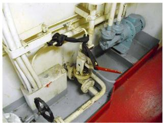
Quick Closing Valve held open with strop
