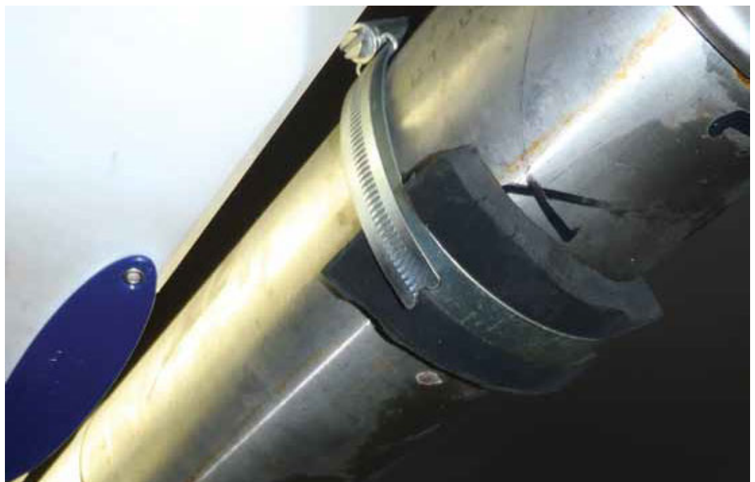
^ Rubber insertion and hose clip
