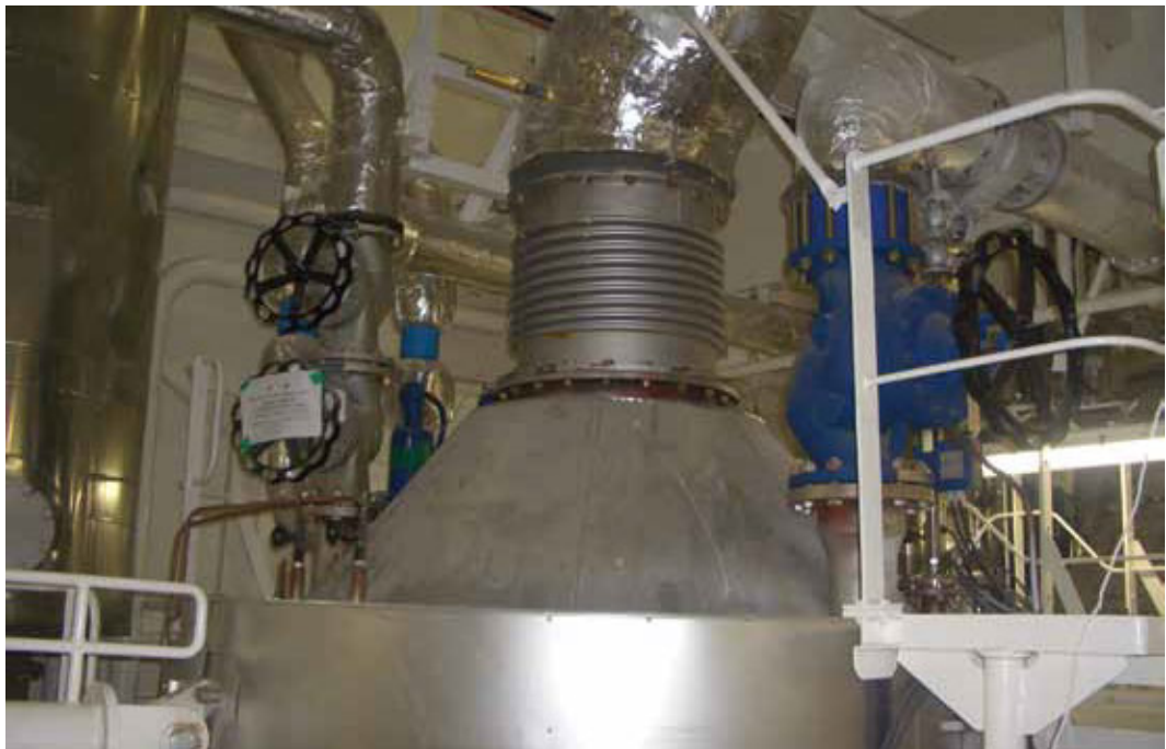
^ Exhaust pipe compensators (bellows)
