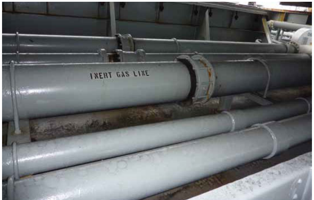
^ Typical inert gas piping
