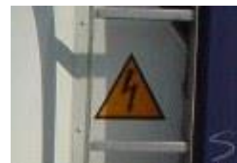
Figure 8.5 Overhead warning sign
