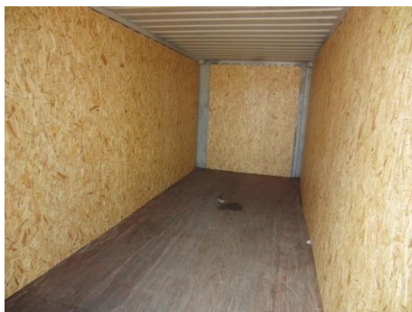
Figure 7.53 Lining a 40-foot container with chipboard panels
