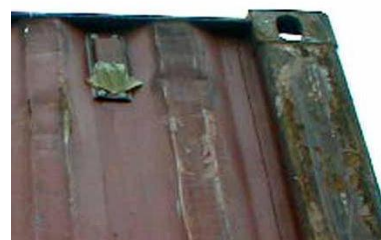
Figure 5.20 Vent tapped over
