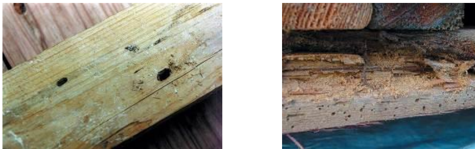
Figure 6.13 Wood frass from boring insect
